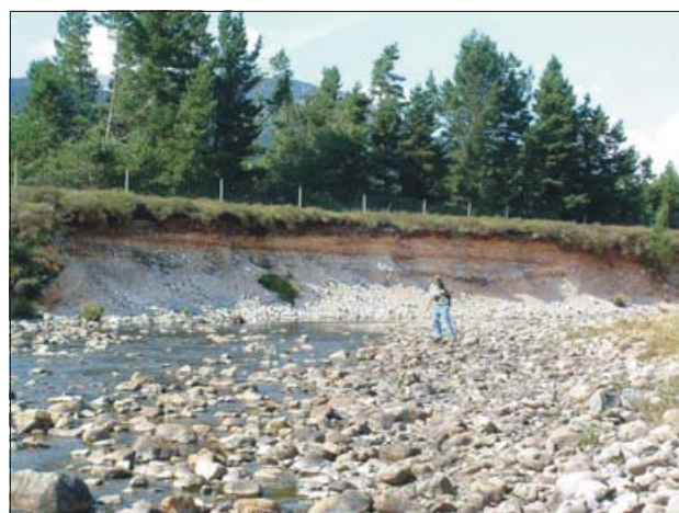
Bank collapse in the Fionn abhainn at NGR 1956 8447. There are several alternative methods for stabilising erosion scars of this sort ( Peter Cunningham )
